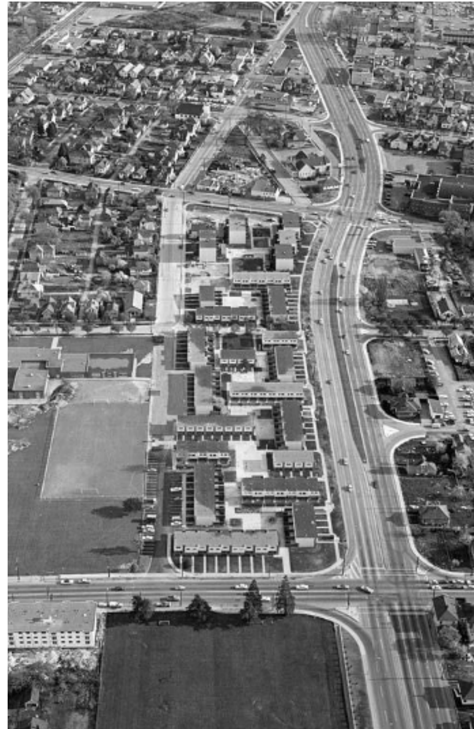
1970's Oblique Aerial view of Blanshard Street looking south towards
